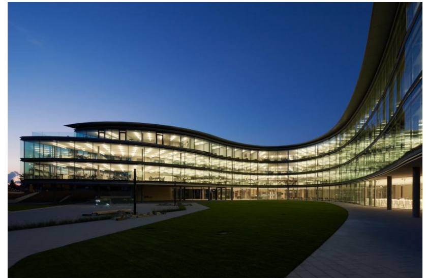
Building technology: Swarovski HQ – Zürich
